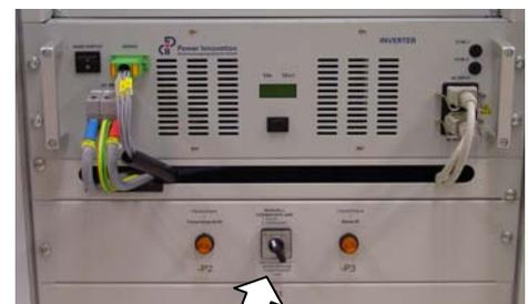
4. Turn the bypass switch into position 2 (Bypassed).
