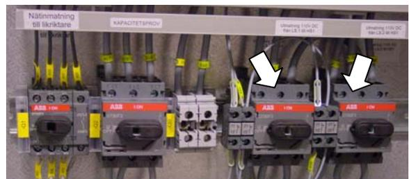
Normally, infeed from battery A is controlled by the left breaker and infeed from battery B by the right breaker.
