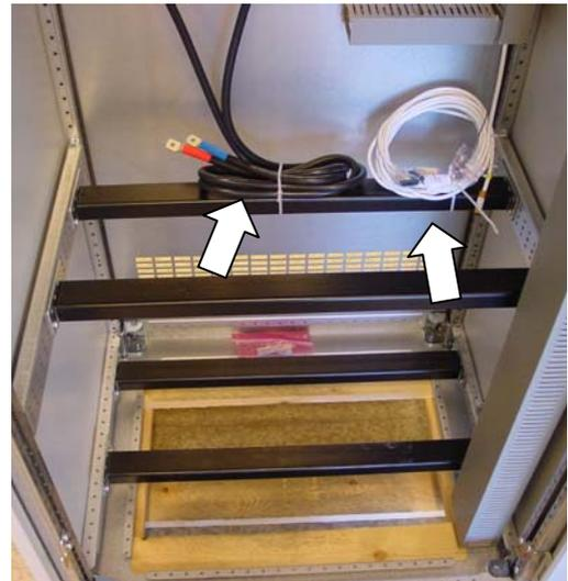
Connect the enclosed short-circuit protected cable set for mid voltage measurement according to the *Manual for Monitoring unit type PCM2*. A spade terminal for mounting on battery bolt M6 and M8 is enclosed. The point of connection should be as close to the electrical midpoint of the battery as possible. In case of an uneven number of cells, the exact midpoint is physical unreachable. Preferably, the battery pole on the minus side of the midpoint is chosen.
