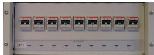
The left short side of the board has a folding plastic case that holds a fuse list. The list is normally left empty by delivery. For a template file in Excel-format, please contact KraftPowercon Sweden AB.
