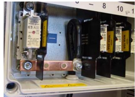
Plastic box for up to eight fuse ways (see the lower picture): Pull in the battery cable through the gland of the box. Provide the cable end with a tube cable lug suitable for an M10 bolt. Screw the cable lug on to the connector plate of the busbar shown on the lower picture.
