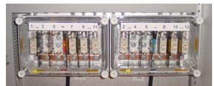
By removal of all fuses in the battery fuse board and switching off the mains breaker the cubicle can be put into a neutral condition, apart from the batteries themselves, the battery fuse box copper bar and a possible bypass mains for inverter.
