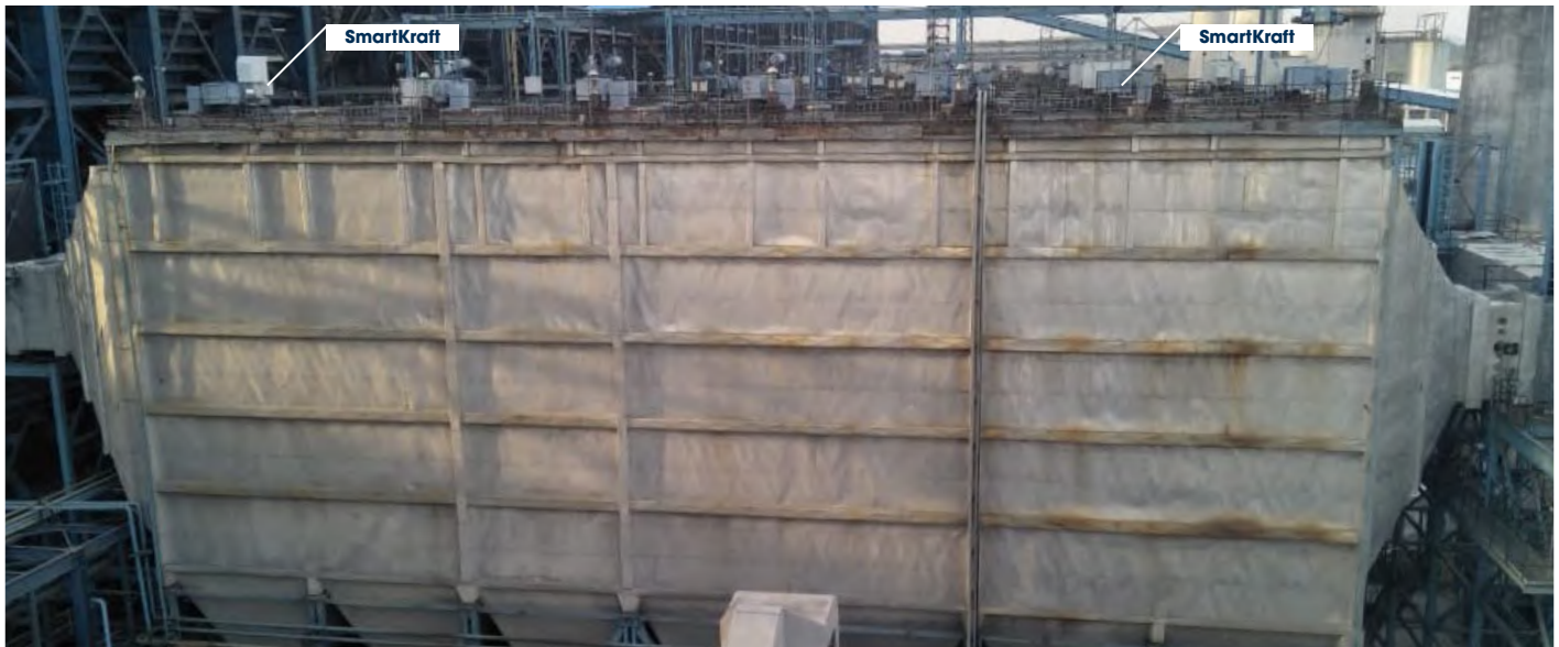
Figure 7: ESP view after PulseKraft® and SmartKraft installation are done.
