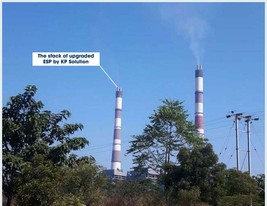
Figure 8: the obvious result of visible smoke at the stacks compared between the ESP which is upgraded by Kraftpowercon ESP solution and the one which is not
